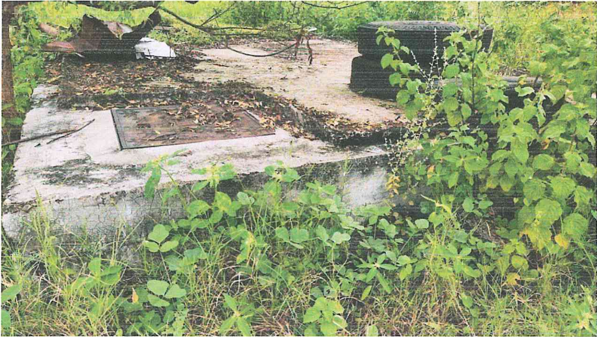
Rain harvesting pit beside B-block.
