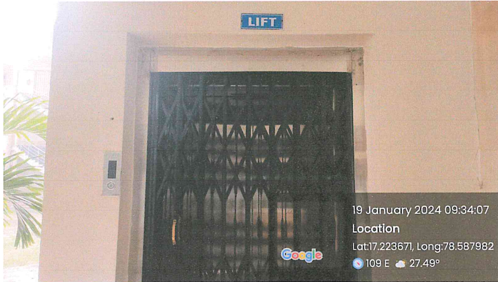
Lift at Block-A
